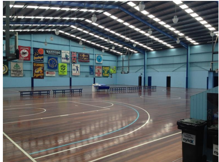
Image 4: skylight installation complete
